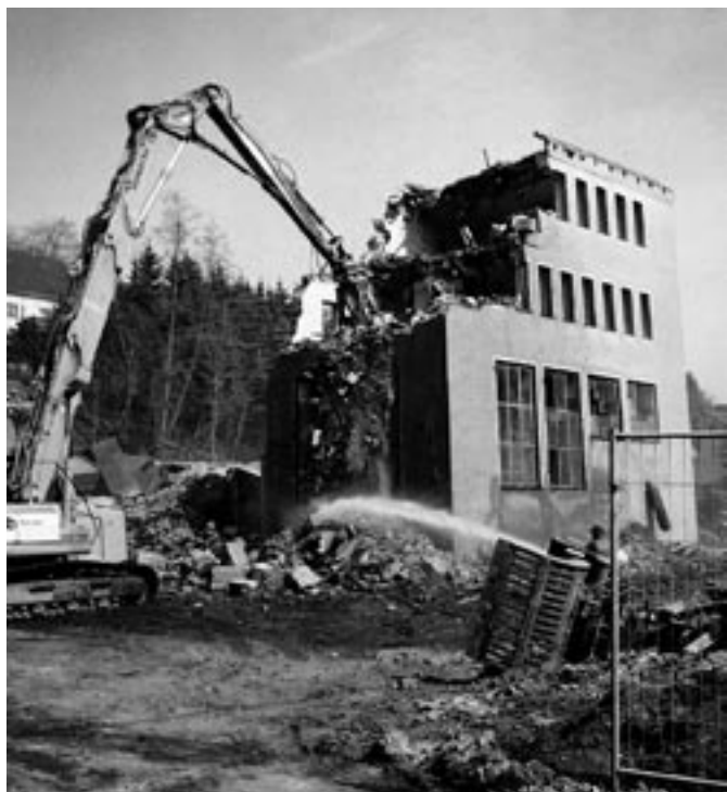
Abriss Sudhaus am 1. April 2008
